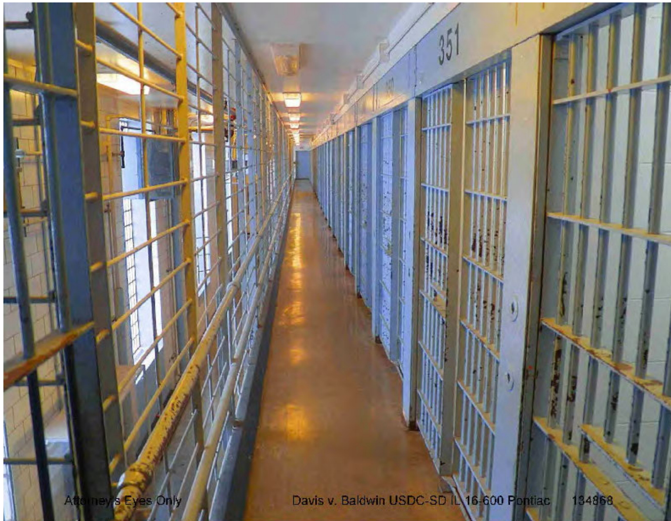
Pontiac Correctional Center - South Mental second floor gallery
