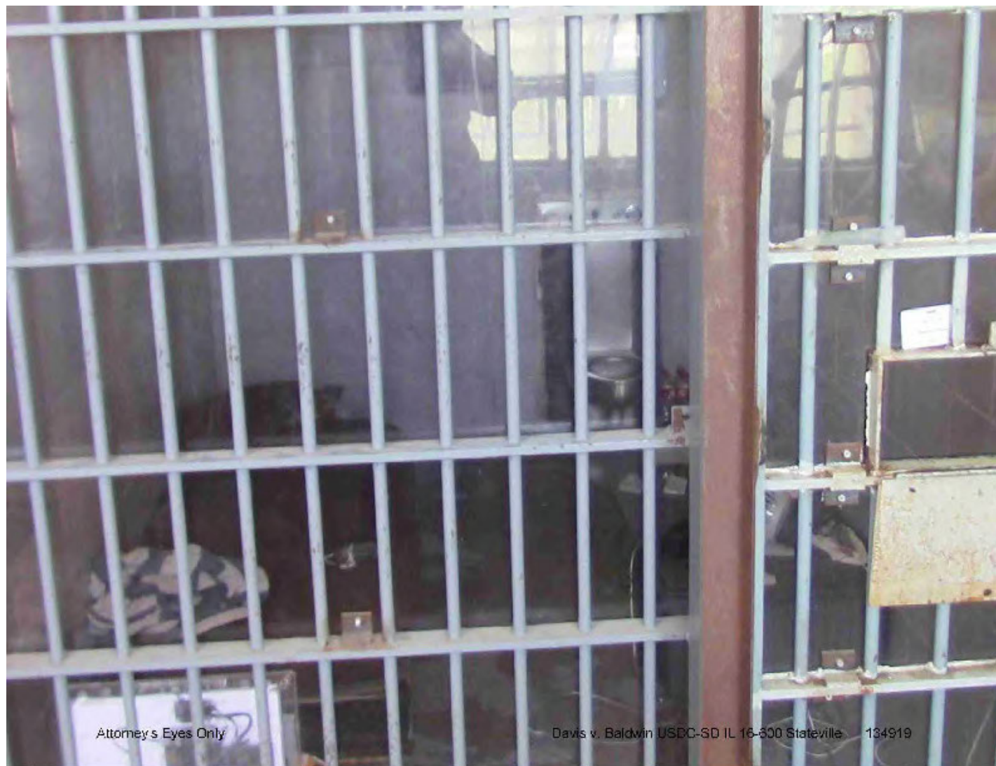
Stateville Correctional Center - Picture of cell door covered completely with Plexiglass
