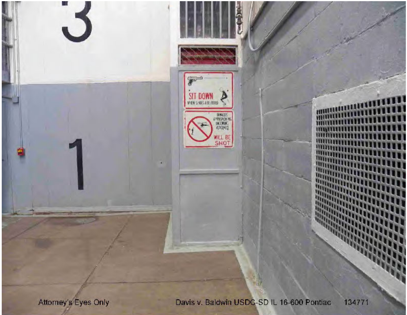
Pontiac Correctional Center - Exterior view of West House cells
