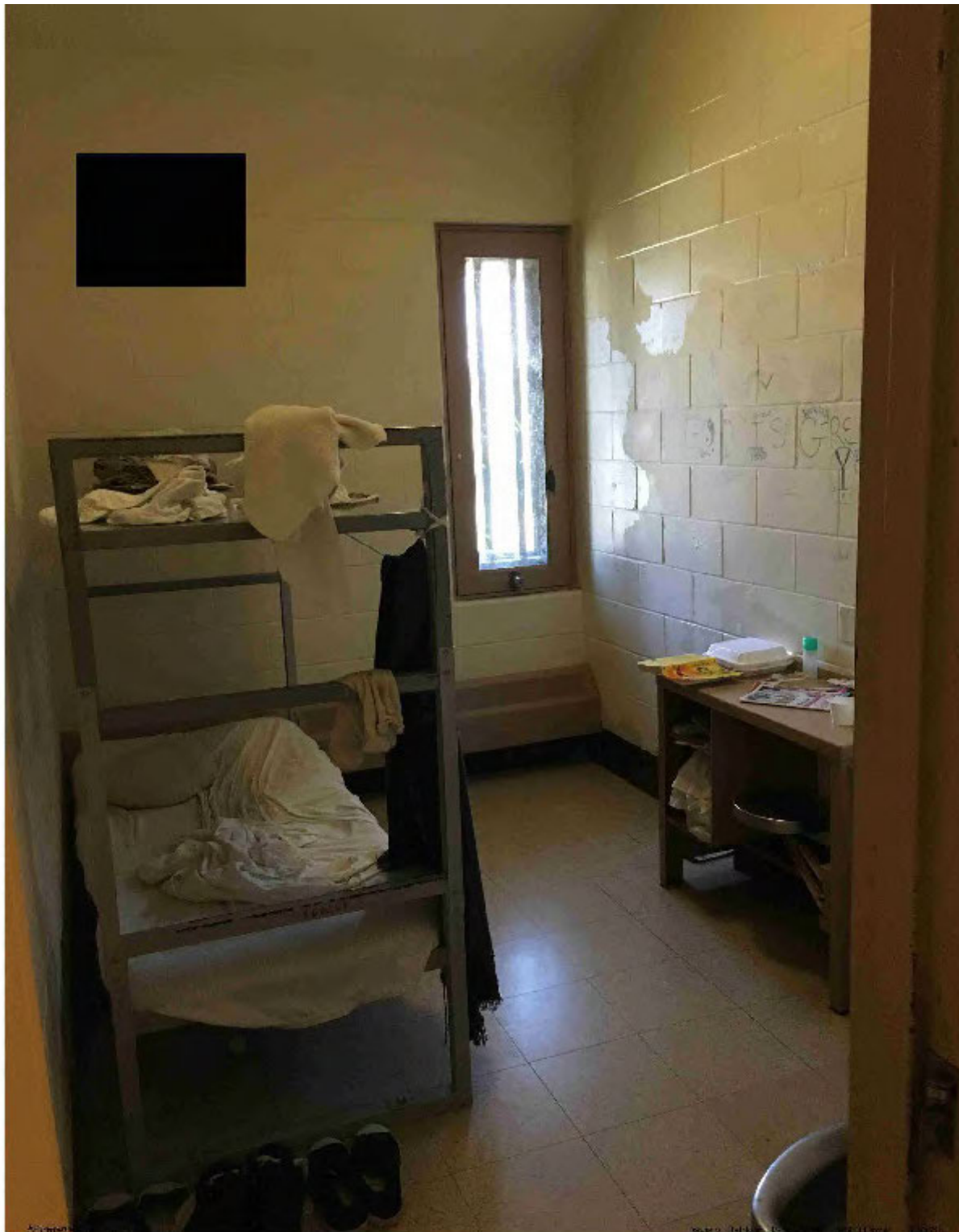
Dixon Correctional Center - Cell in mainline restrictive housing unit
