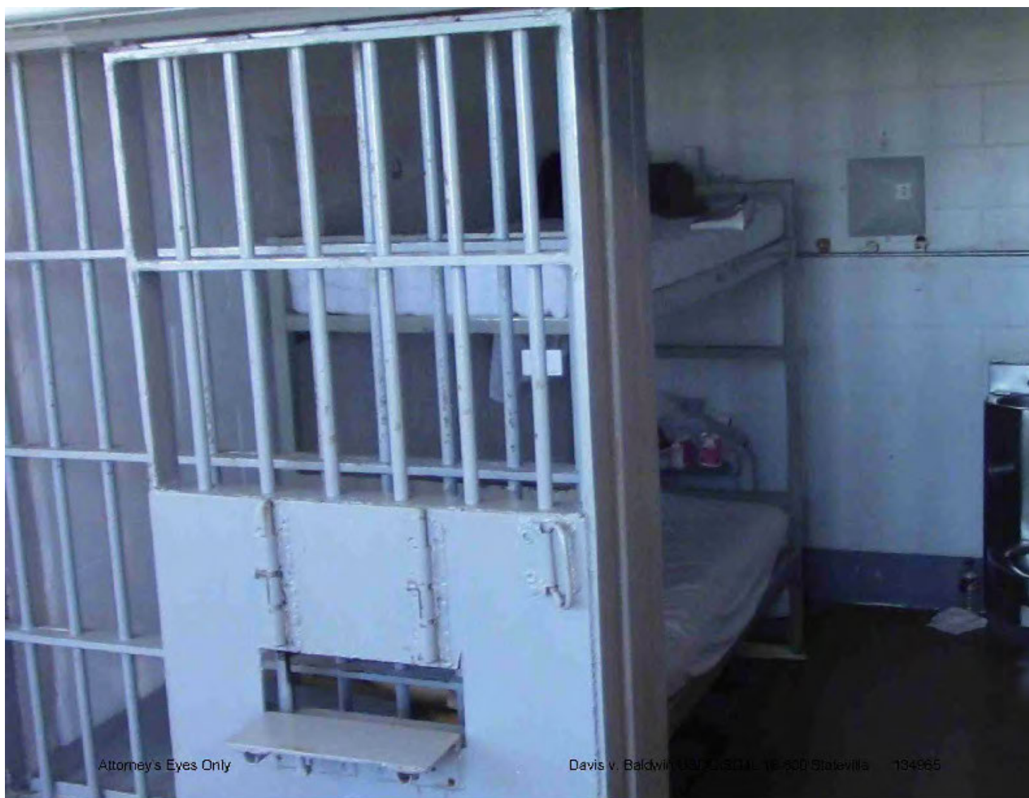
Stateville Correctional Center - Picture of open barred cell in Stateville's X House
